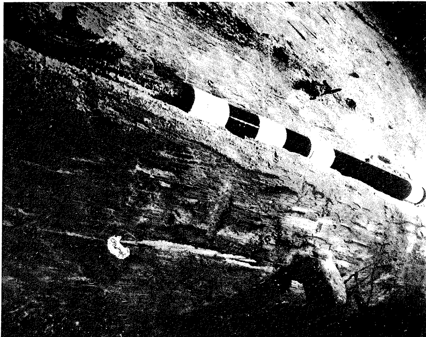
Fig. 14 Photograph of the false keel showing false keel fastenings.
