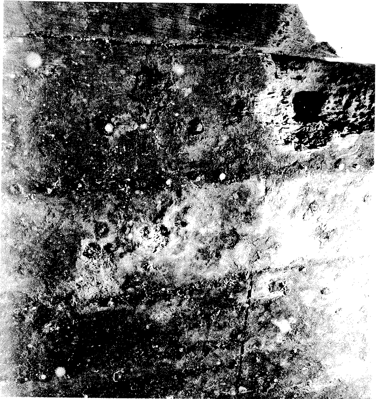
Fig. 9 Photograph showing outer planking with rows of copper sheathing tacks clearly visible.
